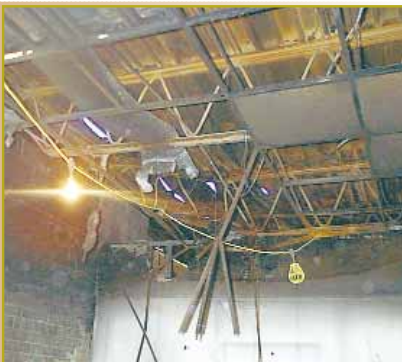
Credit union ceiling—and roof—will be totally replaced
