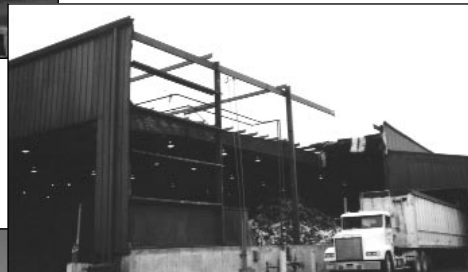
Allen Keith employees replaced steel beams, electrical wiring, lighting, roof and siding material shown in these before, during and after photos.
